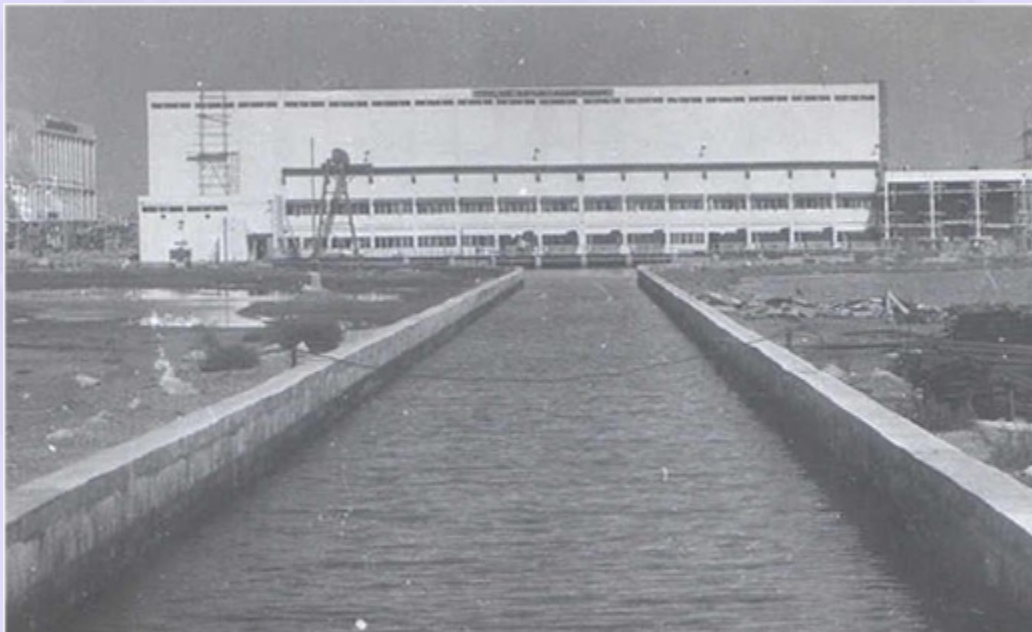
Cooling water intake channel, Tuticorin View towards the Power Station
