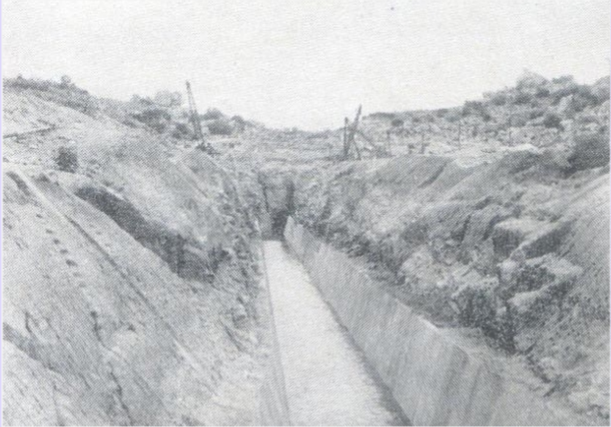
Canal piercing through a hill range by a tunnel, Tungabhadra Project
