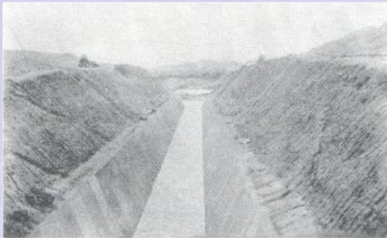
Lined Canal, Tungabhadra
