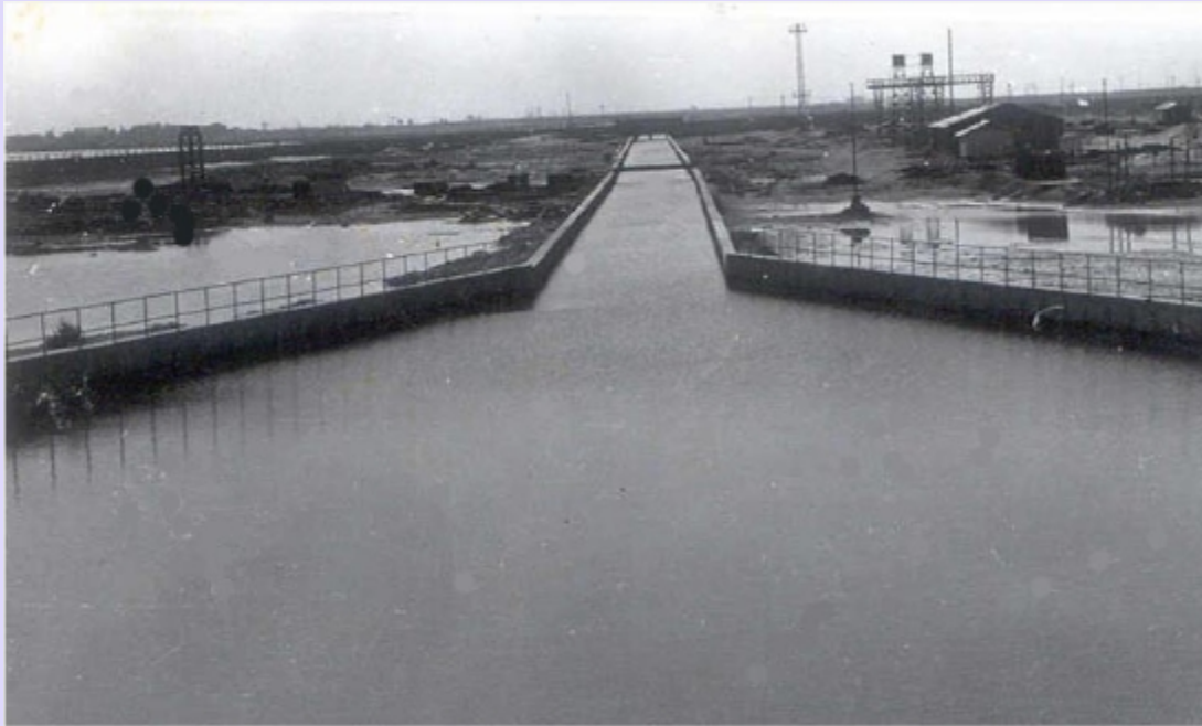
Intake Canal - View towards the Sea, Tuticorin
