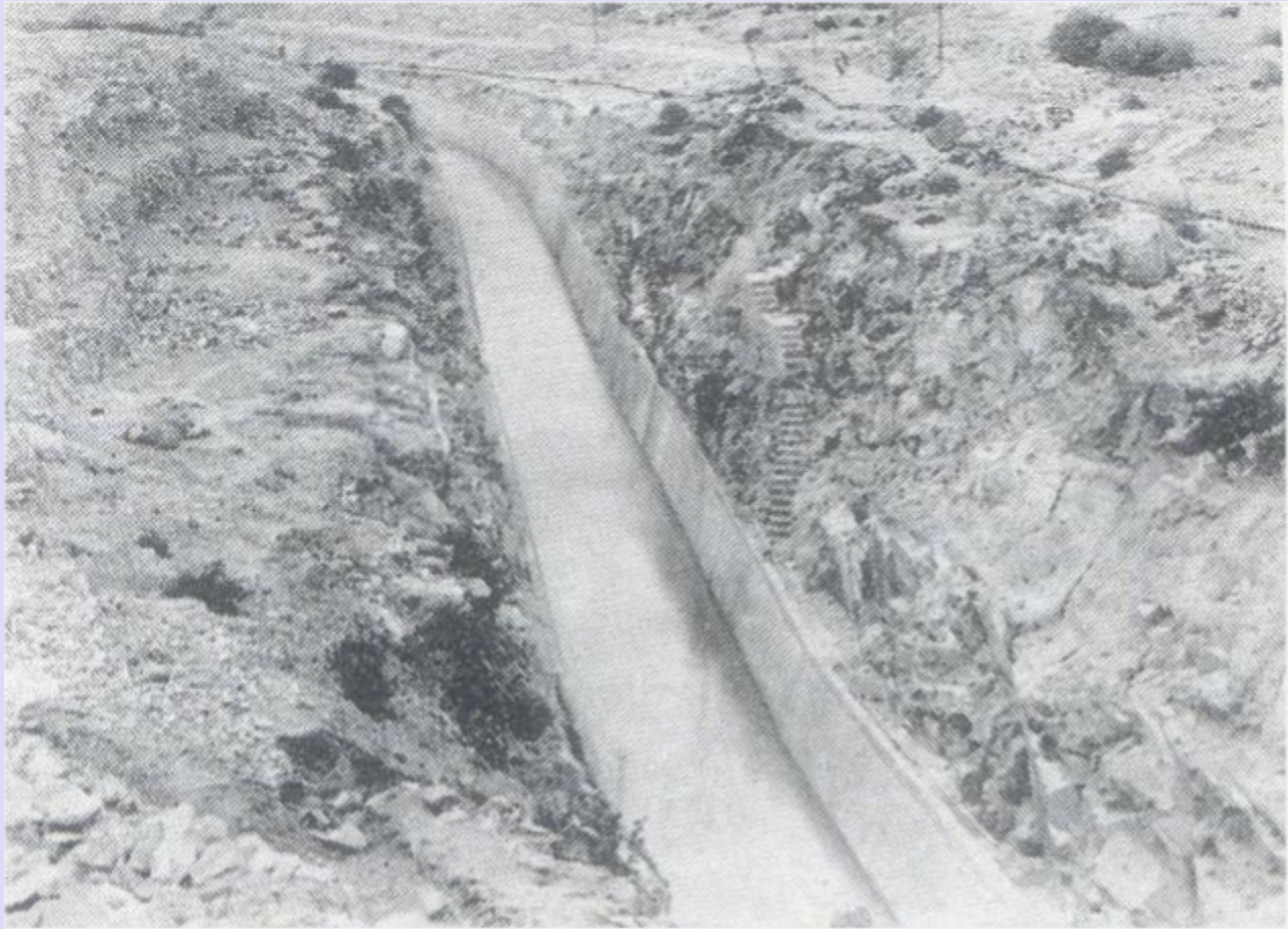
A lined canal, Tungabhadra Project
